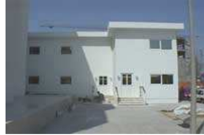
New Office of the Head of Minor Projects (Abu Dhabi PWD). Plywood roof and cement board walls
