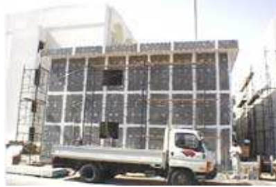
New Office of the Head of Minor Projects (Abu Dhabi PWD). Plywood roof and cement board walls
