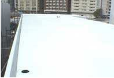
New Office of the Head of Minor Projects (Abu Dhabi PWD). Plywood roof and cement board walls
