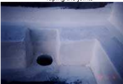
Taping the joints
