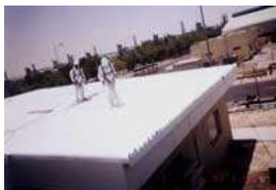
Dubai Training Workshop – asbestos roof coated with Thermo-Shield® Roof Coat
